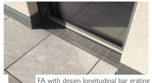
Slot top with drainage-slots for drainage of the second level
