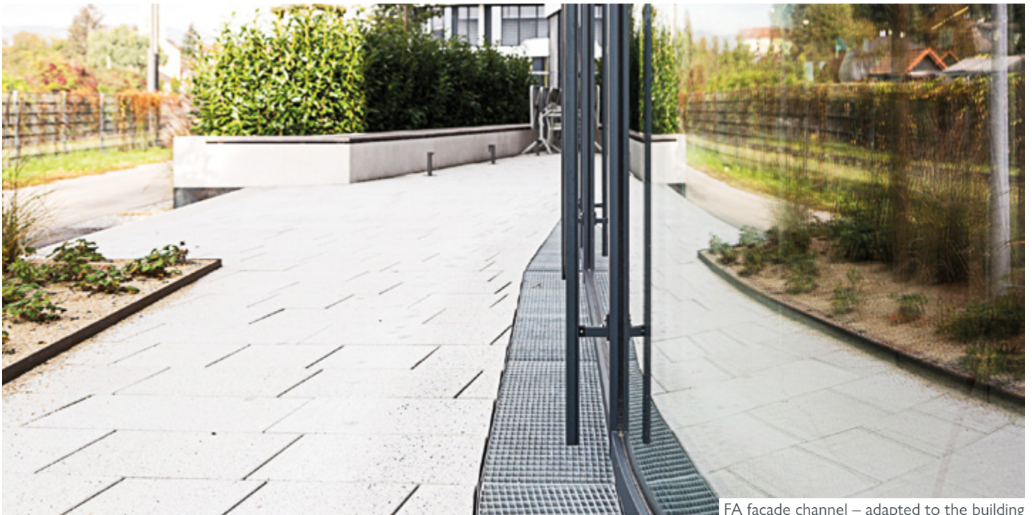
FA facade channel – adapted to the building
