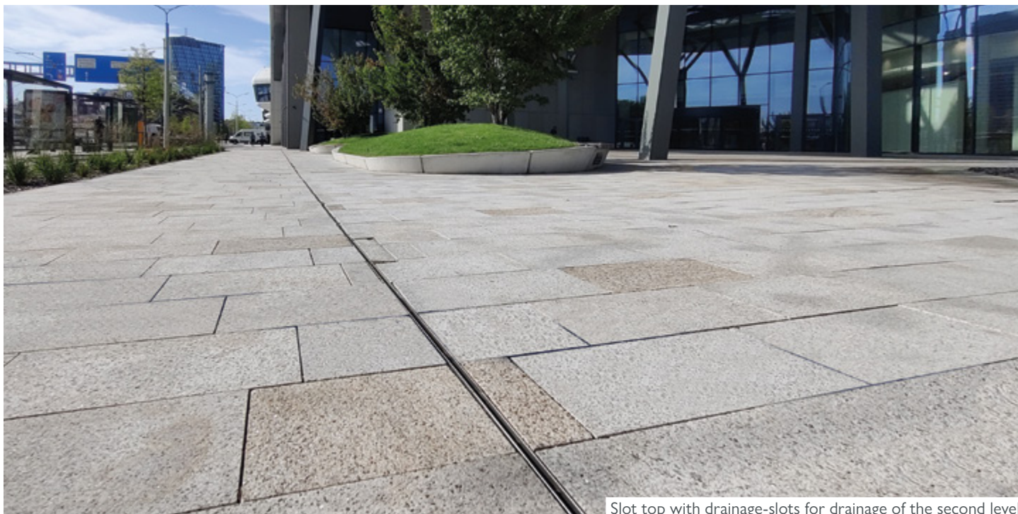
Slot top with drainage-slots for drainage of the second level
