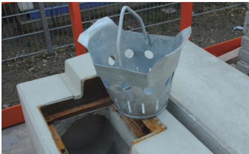
Installed sump unit
