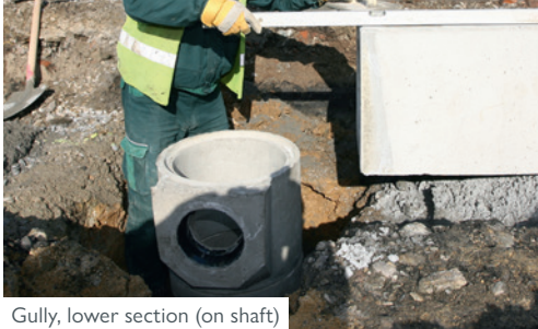
Gully, lower section (on shaft)
